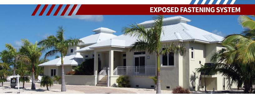
The 5V Crimp roof panel offers an ideal old-time, residential appearance. 5V Crimp is also an aesthetically-pleasing solution for light commercial applications. The 5V Crimp panels require a solid roof deck with a waterproof membrane.
